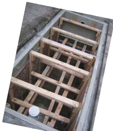
A well braced tank
